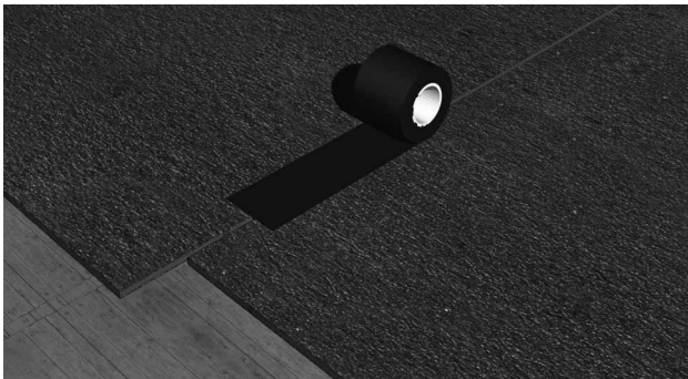
Butt-joint Impact Mat 300 and seal with 75mm or 100mm tape.
